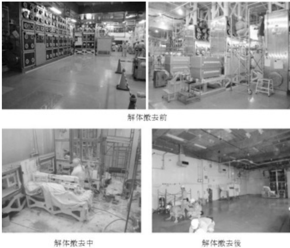
Fig. 7 Progress of dismantling operations for GB (the second decommissioning period)
