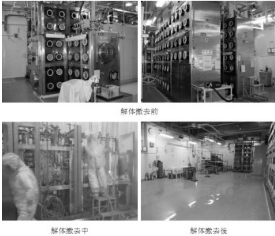
Fig. 6 Progress of dismantling operations for GB (the first decommissioning period)
