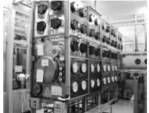
Fig. 2 Typical GB for fuel fabrication equipment
