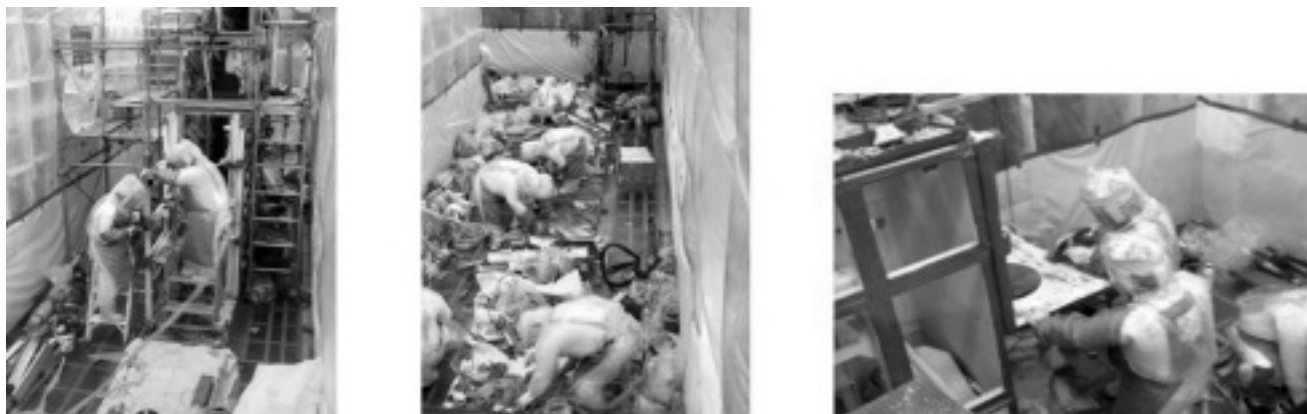
Fig. 4 Dismantling operations conducted by workers wearing air-feed suits
