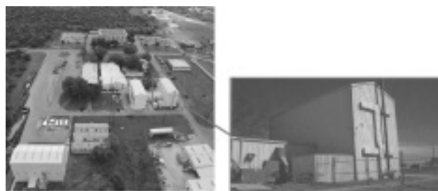
Fig. 7 Underwater demonstration test (IHI Southwest Technologies: San Antonio, Texas USA)
