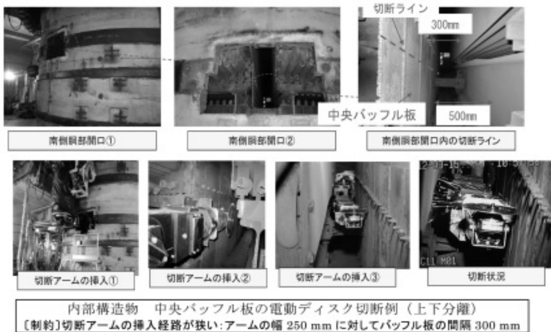
Fig. 1 SRU dismantling in internal narrow area
